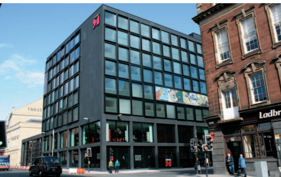
More and more hotels will move all their IT functions off-site. The Glasgow citizenM's PMS is managed from a data centre in Munich.
